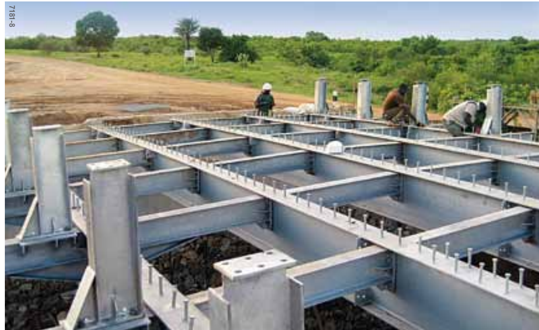
Far Left: Continuous composite beam bridge, Maphutsaneng Bridge, on the Mophales Hoek-Mekaling road, Lesotho - Africa.
