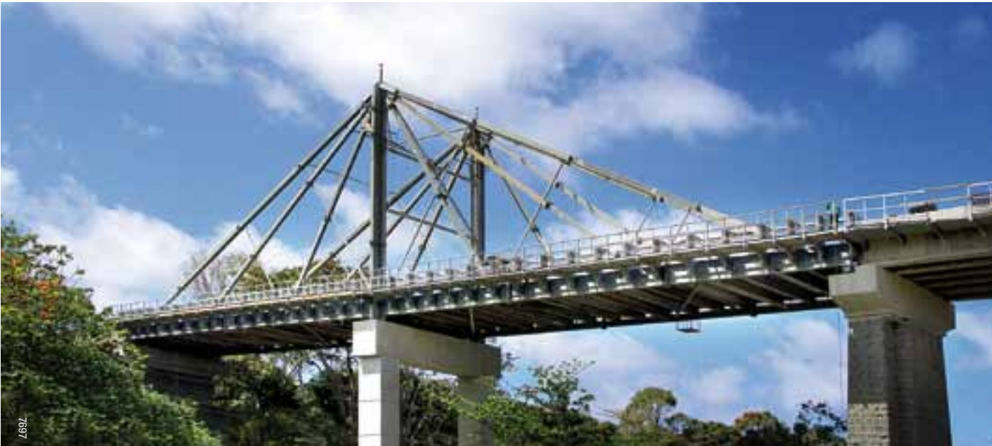
64.8m REIDsteel bridge in Mauritius. Contractors BCE Erection by JTec
