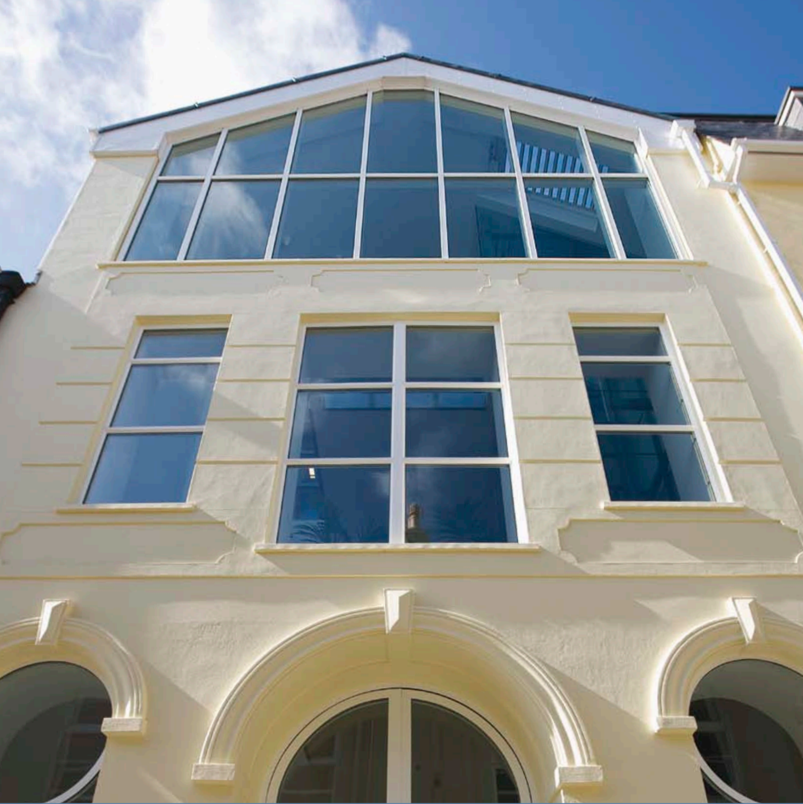
Above: Guernsey Glass (6960) building with fire rated glazing fitted.
