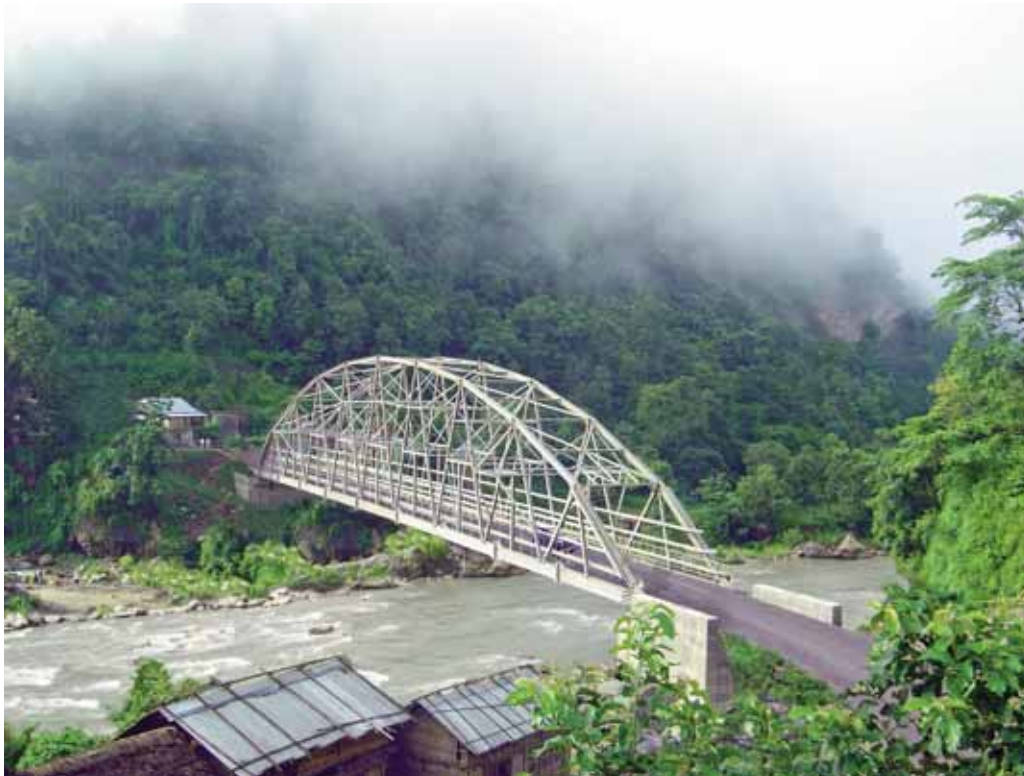
Figure 4. The finished bridge. Designer Peter Mrozinski, Draughtsman Kevin Williams, both of REIDSteel.
